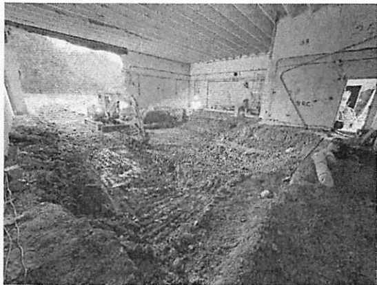
Figure 4. Hot Cell Post-Demolition
