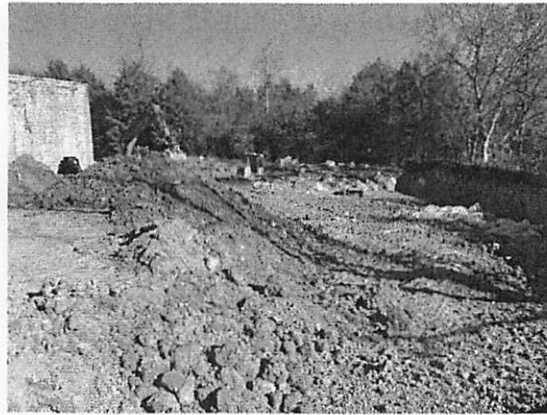
Figure 2. Mounded Area Post-Excavation
