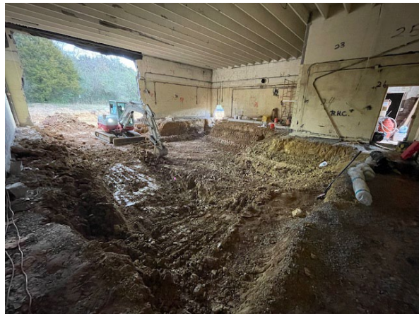
Figure 4. Hot Cell Post-Demolition
