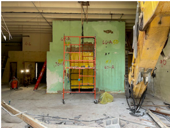
Figure 3. Hot Cell Pre-Demolition
