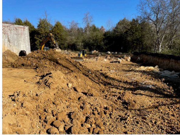
Figure 2. Mounded Area Post-Excavation
