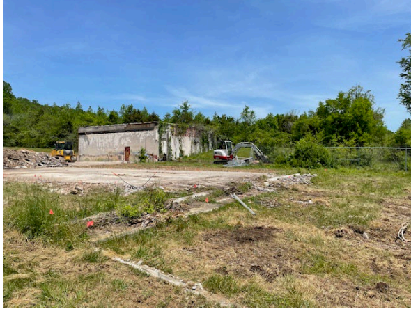
Figure 1. Mounded Area Pre-Excavation
