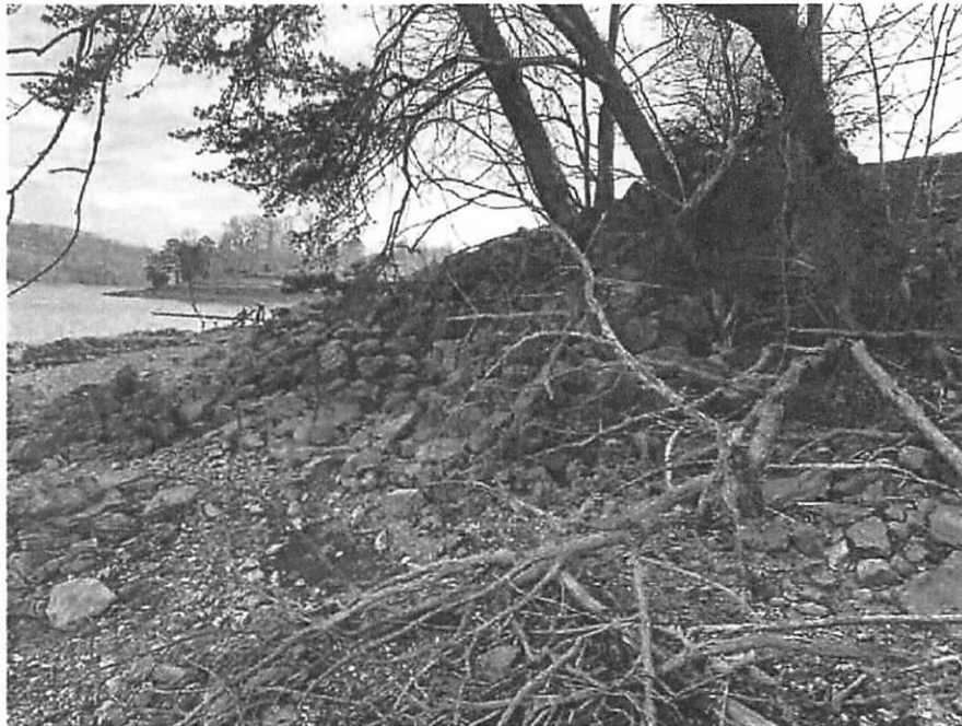
Photo 8: Facing the eastern edge of armor area 1, towards existing rip rap
