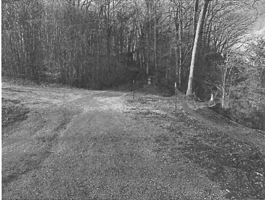
Photo 3: Pedestrian walking path along the eastern edge of armoring area 1
