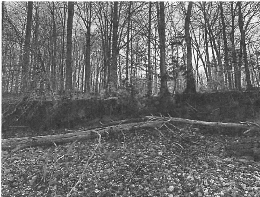
Photo 14: Eroding banks along armoring area 2
