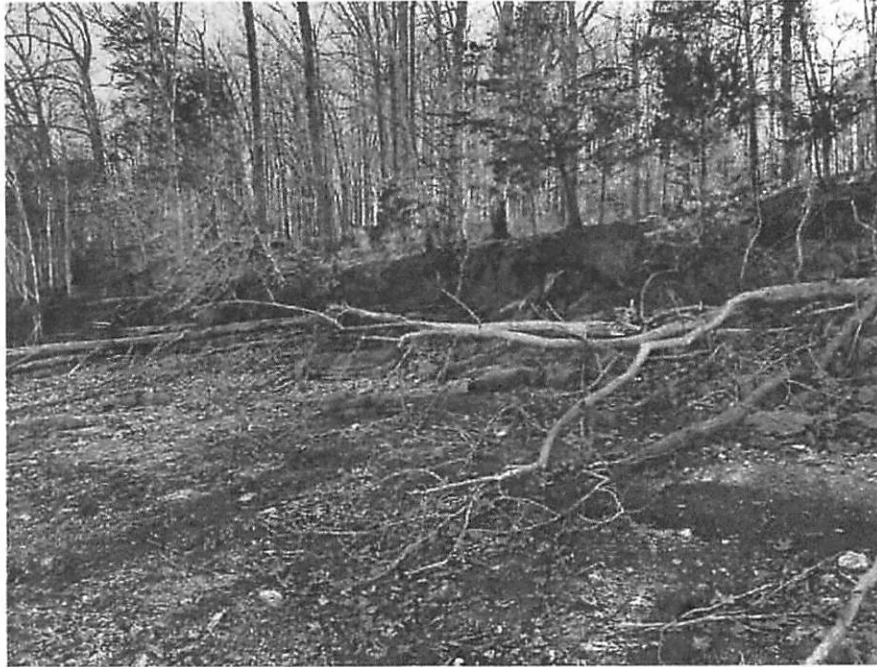
Photo 15: Eroding banks to the north of the campground, approximately 8 feet tall
