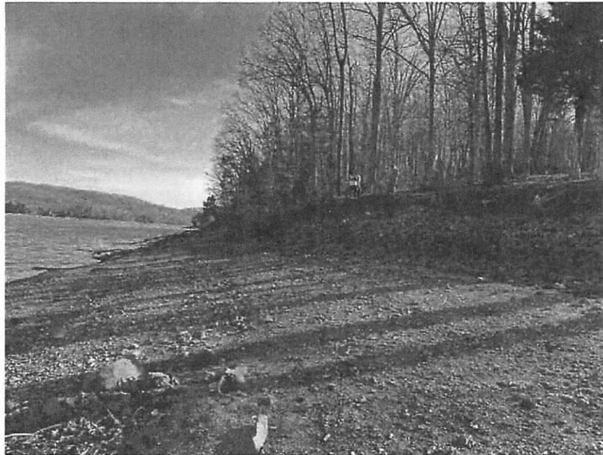
Photo 12: Facing generally north looking towards the eroding stream banks at armor area 2
