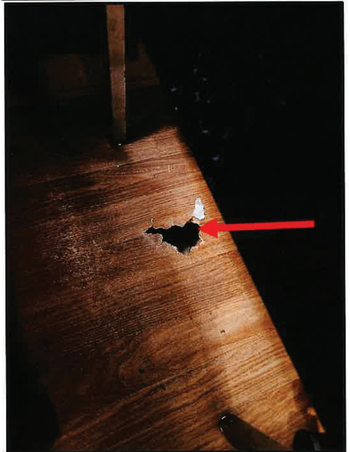
Clinton Station 1: Replace damaged flooring
