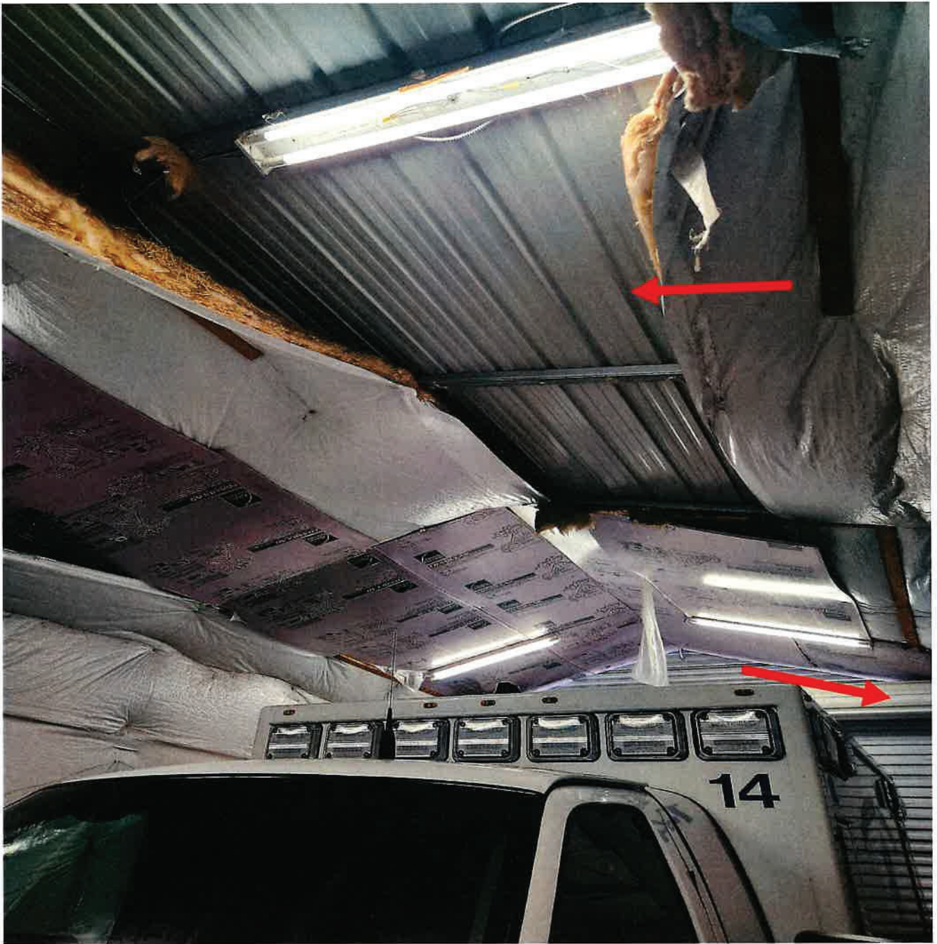
Andersonville Station 6: Replace missing garage insulation, repair non-working garage door.
