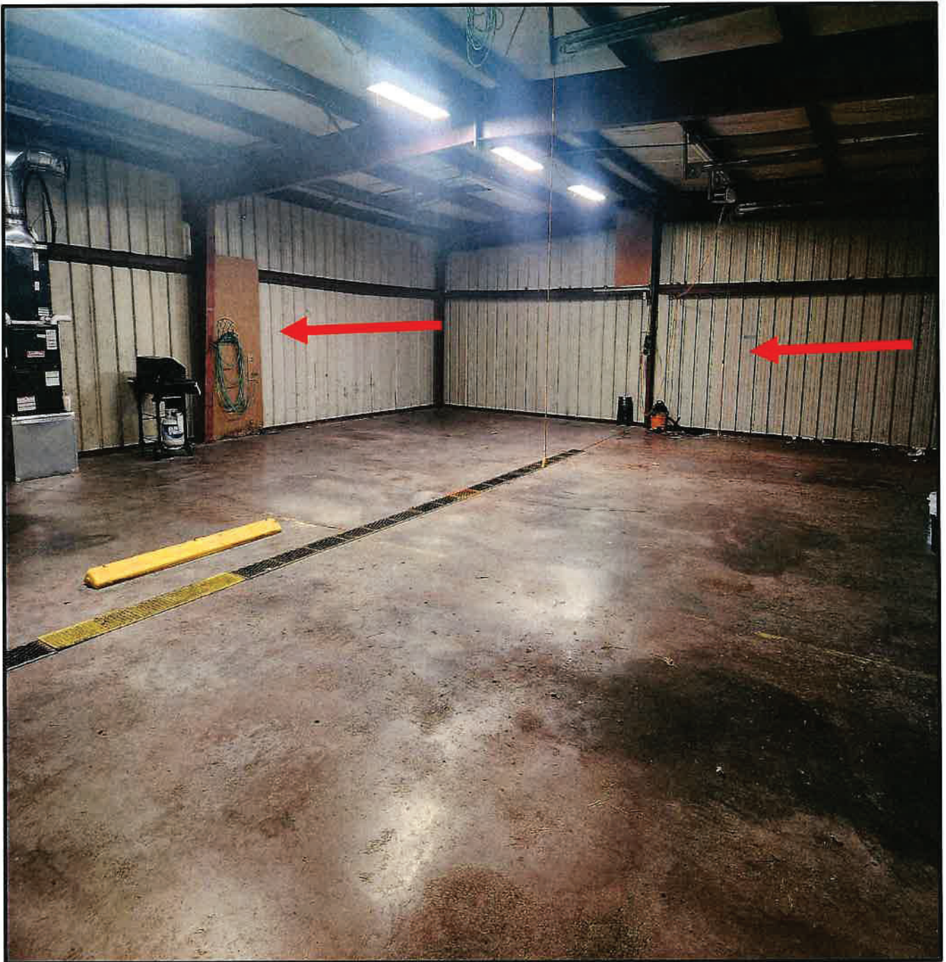
East end Oak Ridge station 5: Add insulation to garage walls
