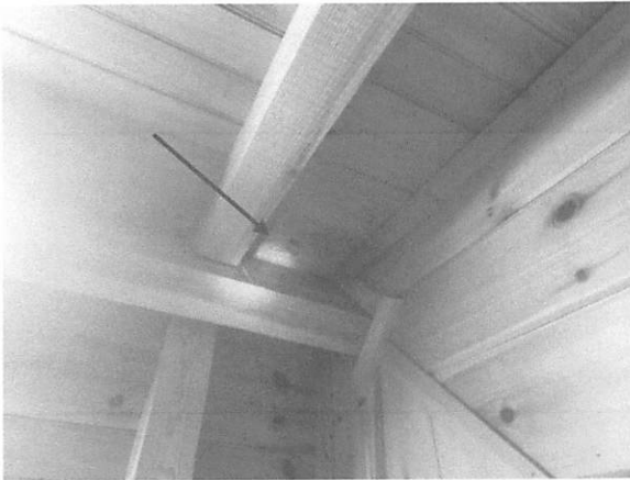
A10 (Suspected mold was observed at the apex of the ceiling in the hallway just outside the affected portion of the ceiling in Stephanie's office.)
