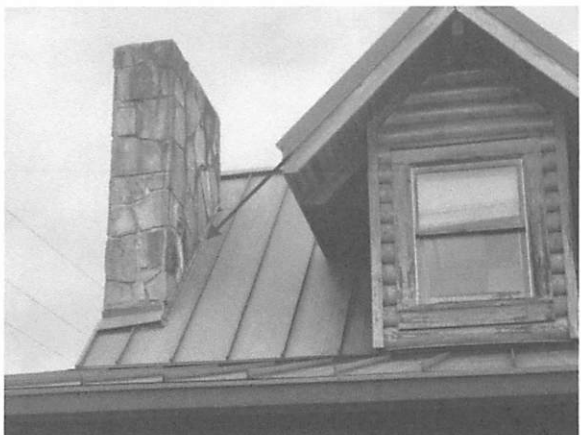
A15 (The chimney on the exterior of the structure appears to be without flashing.)
