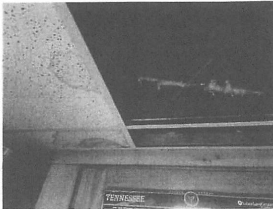
A18 (Water damage was observed in the ceiling of the supply room as a result of roof leaks.)
