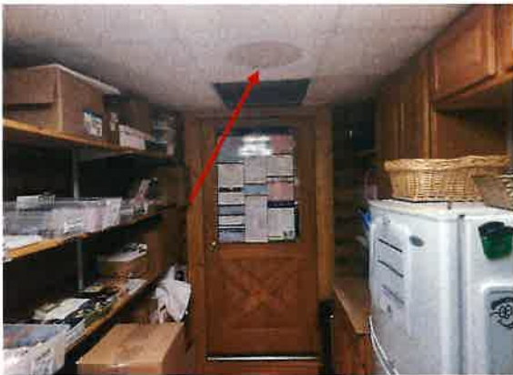
A17 (Water damage was observed in the ceiling of the supply room as a result of roof leaks.)
