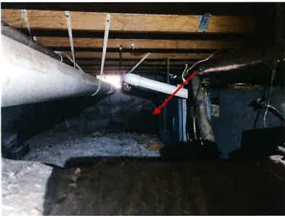
A20 (Dampness observed on the concrete block in the crawlspace just inside the HVAC component pictured in A19.)
