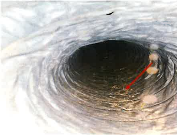
A16 (Accumulations of dust, dirt and debris were observed inside HVAC supply lines.)
