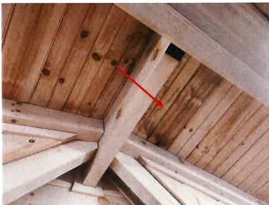
A6 (Water stains and suspected mold were observed at the apex of the ceiling in Stephanie's office.)
