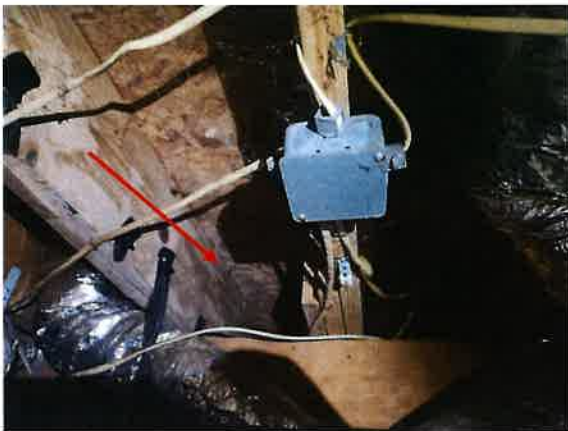
A21 (Water stains were observed on subfloor and floor joists underneath the men's bathroom.)
