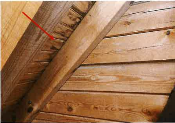
A13 (Water stains were observed in the ceiling of the closet in Teri's office next to the chimney.)
