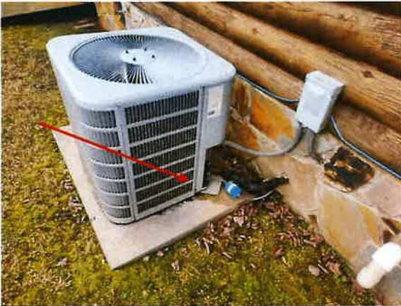
A19 (Water pooling next to the HVAC component just outside of the crawlspace.)
